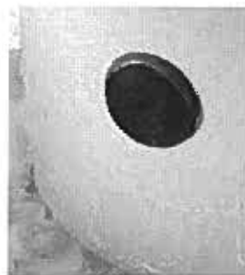
Terset uttak for selvfall
